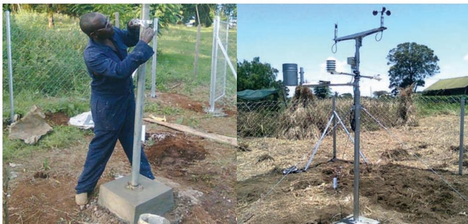
A staff member of the Kenya Meteorological Department installs an automated weather station provided by the project at a farm in Menengai, Nakuru district. On the right is a complete installation.
